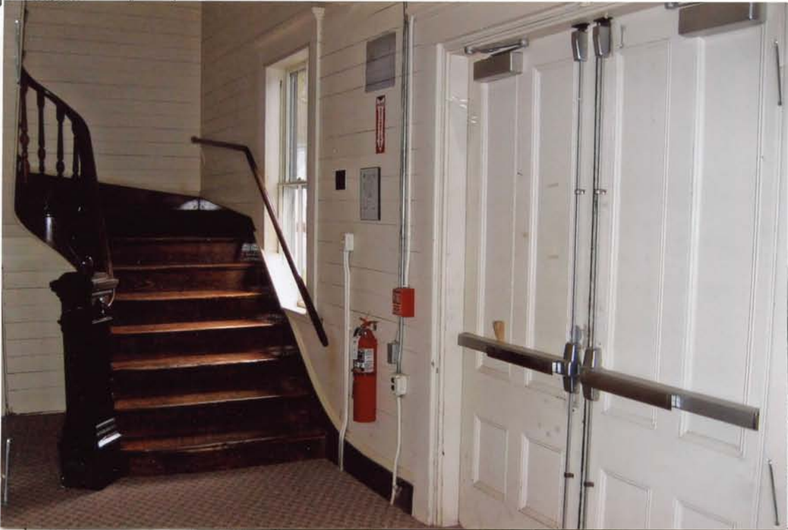
Photo # 10 Description: double door entry, right staircase
