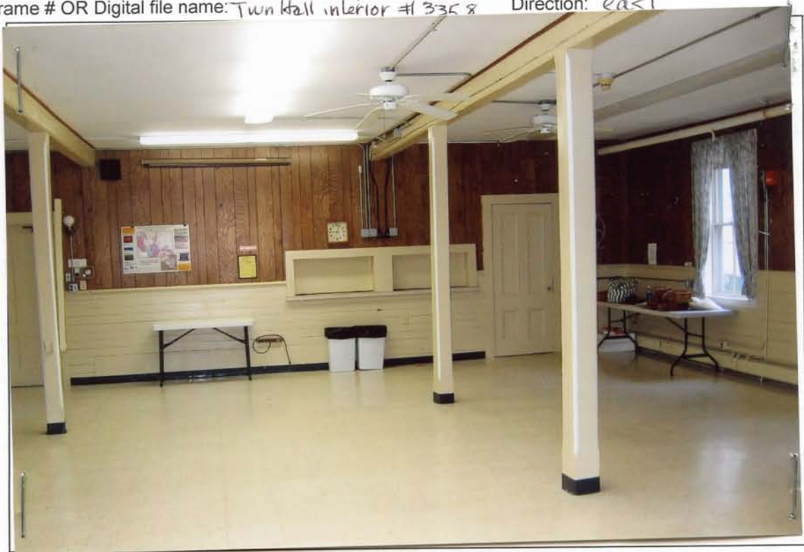
Photo # 13 Description: 1st floor meeting room, facing rear Roll and Frame # OR Digital file name: Town Hall interior #3359 Direction: west
