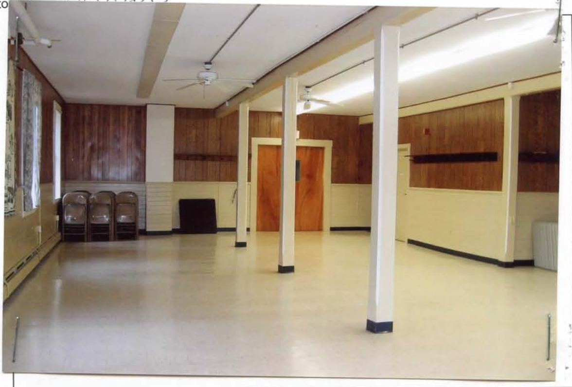
Photo # 12 Description: 1st floor meeting room facing front Roll and Frame # OR Digital file name: Town Hall interior #13358 Direction: east
