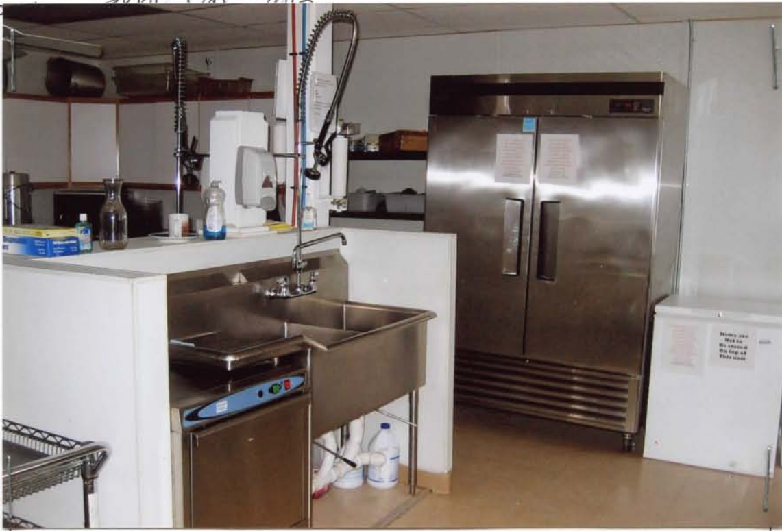
Photo # 14 Description: 1st floor kitchen rear Roll and Frame # OR Digital file name: #3360 Townhall Interior Direction: West west
